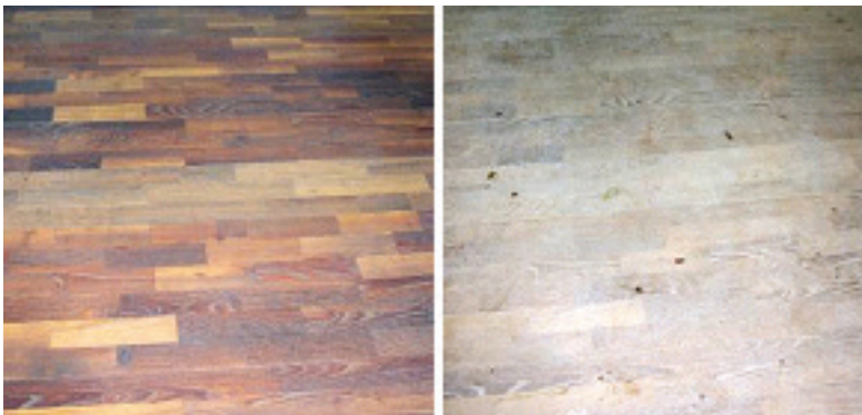
Fig. 7. The original conditions (a) and after exposure (5 year) (b) of the flooring
