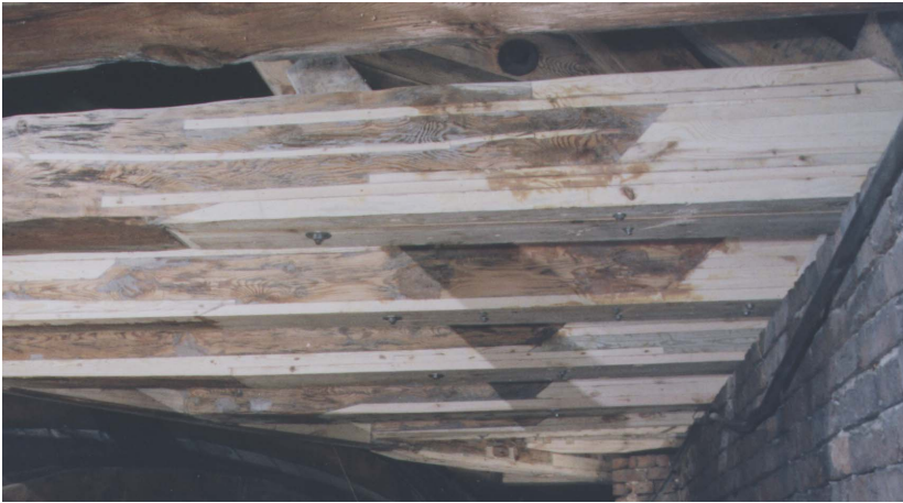
Fig. 6. An example of attic beams reconstruction
